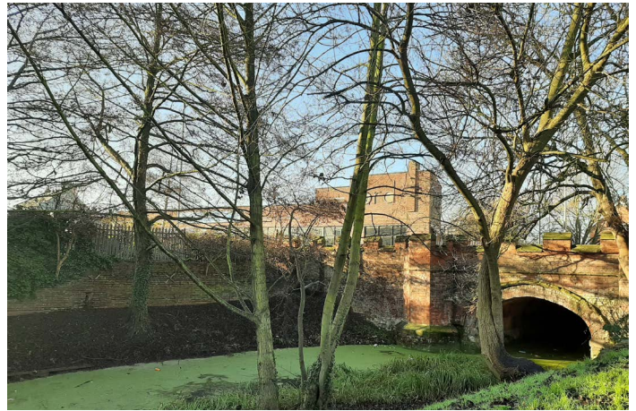
Middleton Stop Drain, Southgates Park
